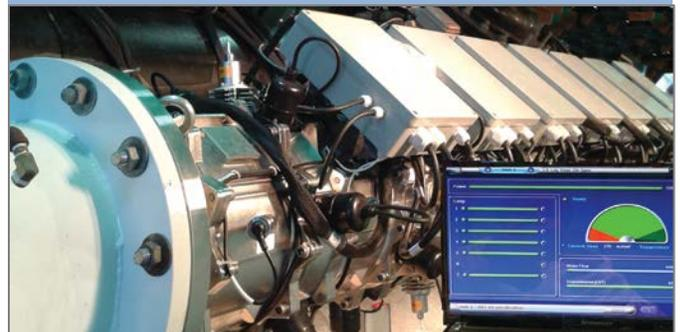
Figure 2: Atlantium RZ300-17 system with monitoring & control software indicating an on-spec 3-log virus UV dose being delivered
