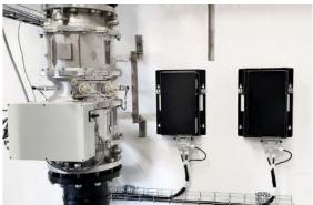
Atlantium's RZ300 systems for IPN protection have been effectively applied in Norway, Scotland, Canada and Chile. The advantage of the wide germicidal wavelength of the Atlantium medium-pressure lamps enables compact and effective installations for water biosecurity.
