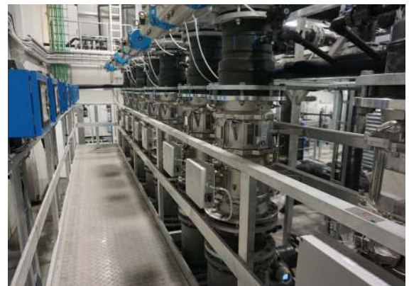
HOD™ UV ensures water biosecurity at the world's first breeding plant for lumpfish at Namdal Rensefisk AS in Flatanger, Norway.
