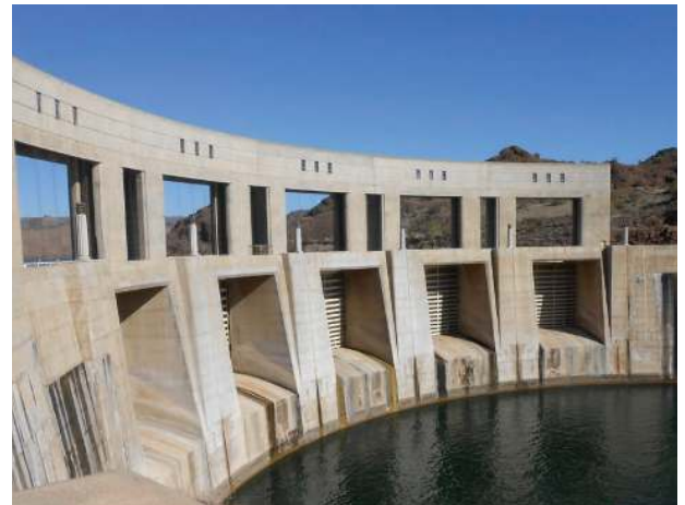
HOD UV systems were installed at Parker Dam to address biofouling concerns from Aquatic Invasive Species (AIS).
