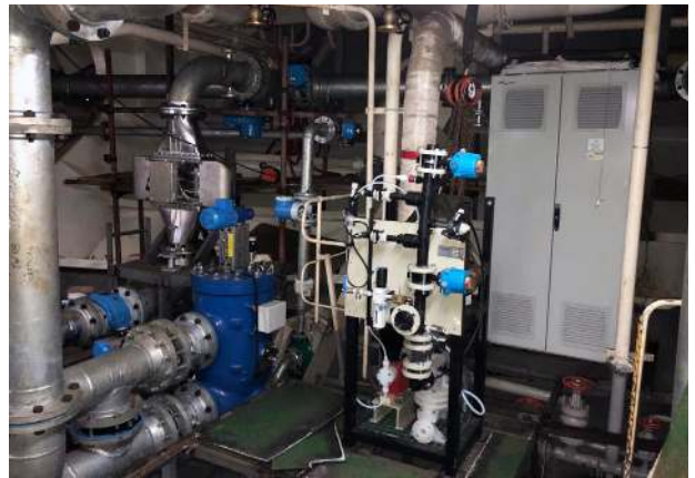
Purestream™ UV-based ballast water management system assures compliance with the strictest inspection processes.
