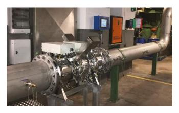
The RZB300-12 with DPM system was installed as a bypass on the existing 300 mm (12") piping and water was returned to the cooling towers, accommodating a flow rate of 250-400 m³/h (1,100-1,761 gpm), as a cost-effective and efficient method of reducing biofilm and providing effective treatment for inactivating Legionella.
