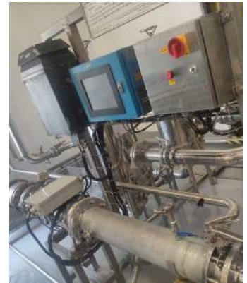
Horizontal system installation in 2023
