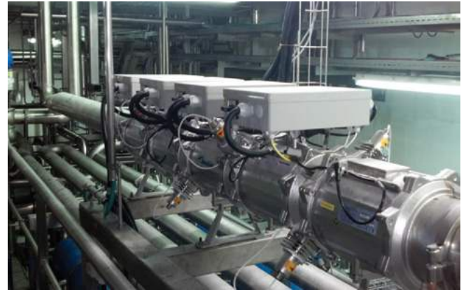
Two parallel Atlantium units treat 85 m 3 /hr of RO permeate
