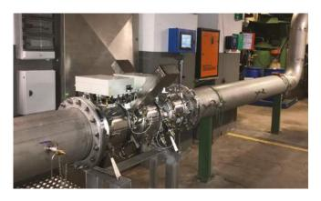
The HOD UV RZB Series was installed as a bypass on the existing 300 mm (12") piping and water was returned to the cooling towers, accommodating a flow rate of 250–400 m³/h (1,100–1,761 gpm), as a cost-effective and efficient method of reducing biofilm and providing effective treatment for inactivating Legionella.
